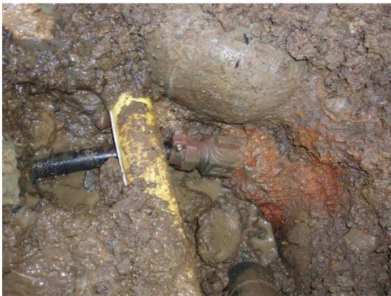
This picture shows just what the Public Works staff encounters when they dig to repair a leak. The light colored pipe is the gas line. The dark line beneath the gas line is the water line that connects to a “saddle” and the main line. As well, you can clearly see the boulders that must be worked around. This particular area has thin walled polyethylene (polyE) distribution lines that are beginning to fail.
